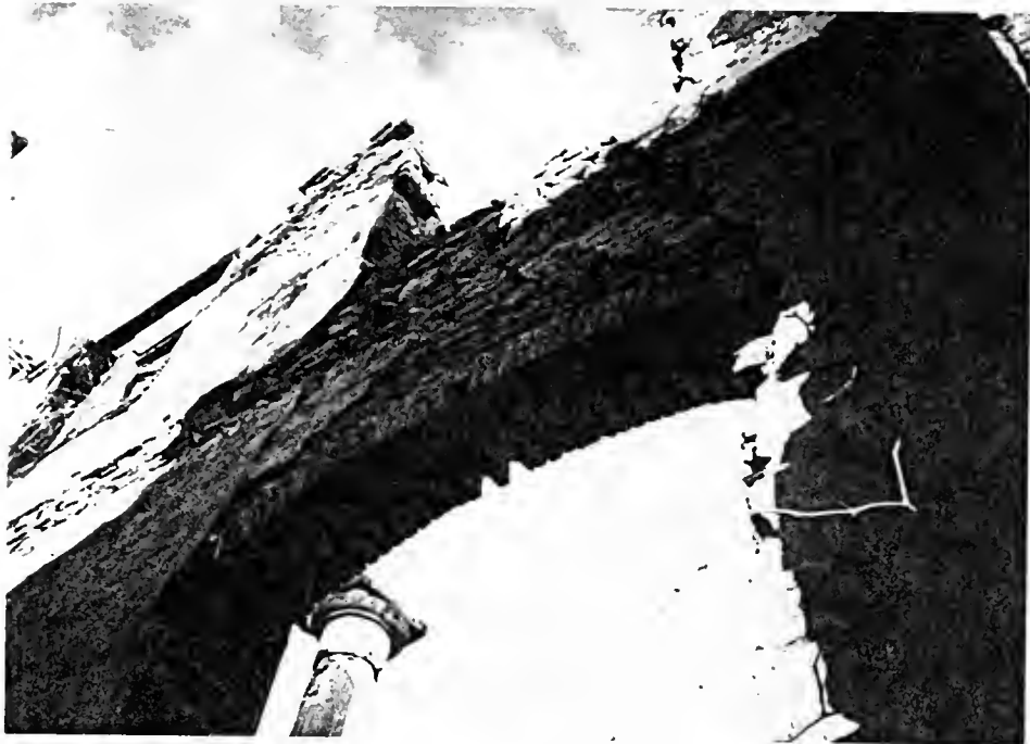
Figure 27: Southernmost arched opening along east elevation, showing loss of stucco and missing bricks within the arch itself
